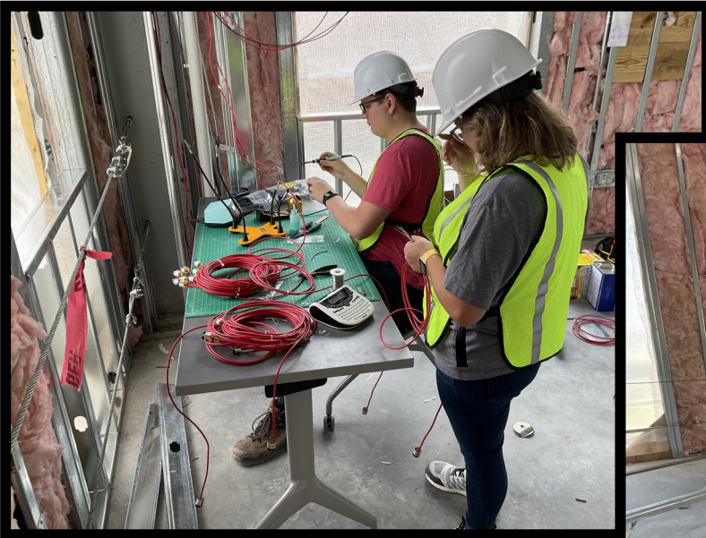
Above and Right: Soldering of spatially distributed sensors in the Ashraf Islam Smart Building.
