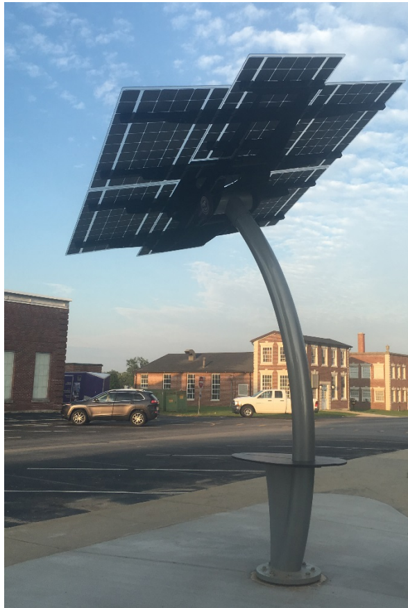
Externally mounted solar panel array for integration with the Smart Grid Laboratory.
