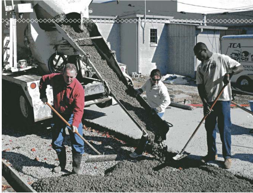
Early TCA Experiments with Self-Compacting Pervious PCC (Photo courtesy of Dr. L.K. Crouch)
