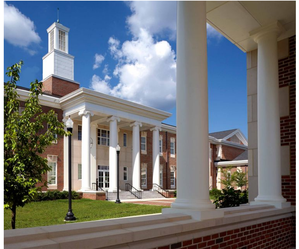
Figure 3.8 Bell Hall courtyard
