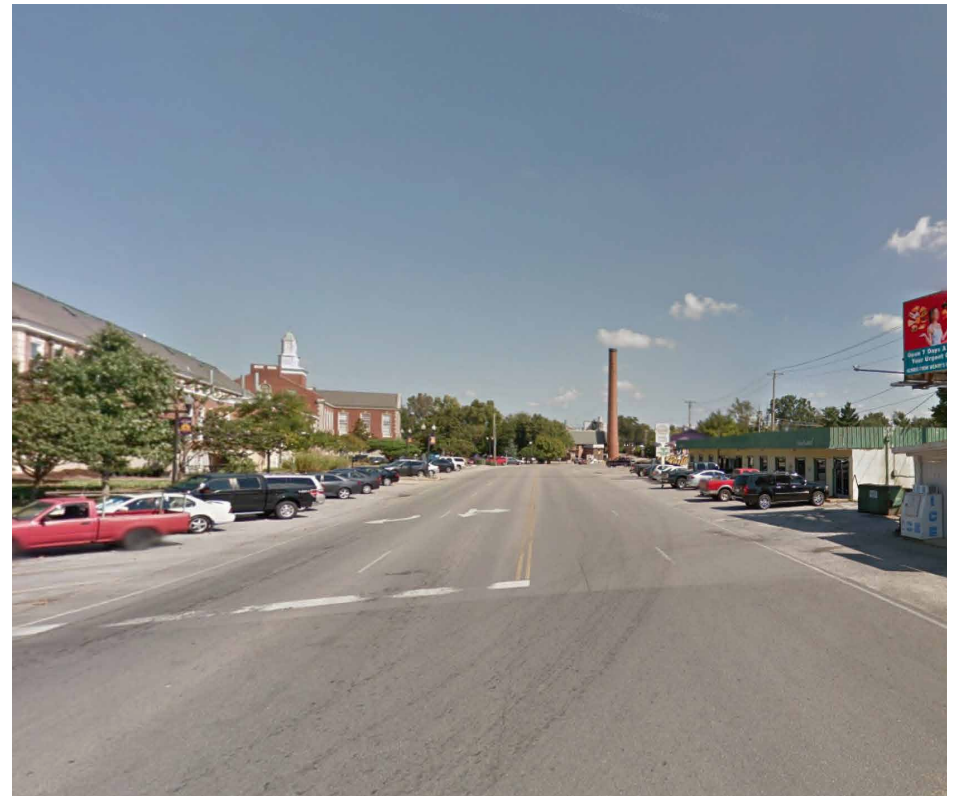
Figure 2.15 Mahler Avenue, north of West 7th Street
