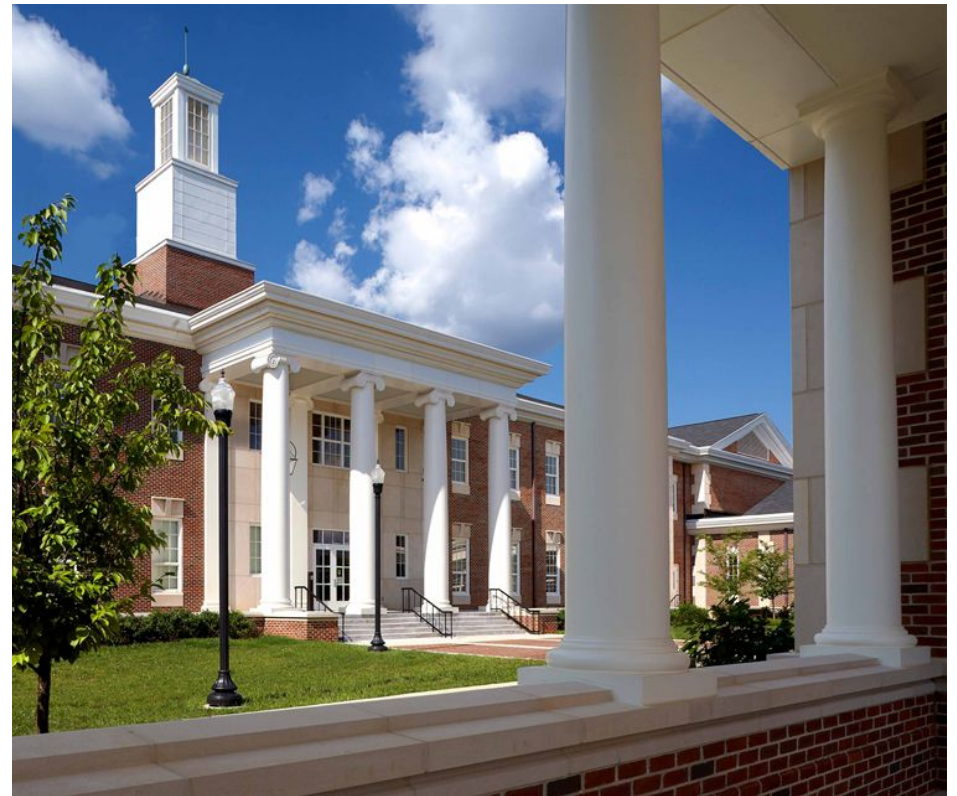
Figure 3.8 Bell Hall courtyard
